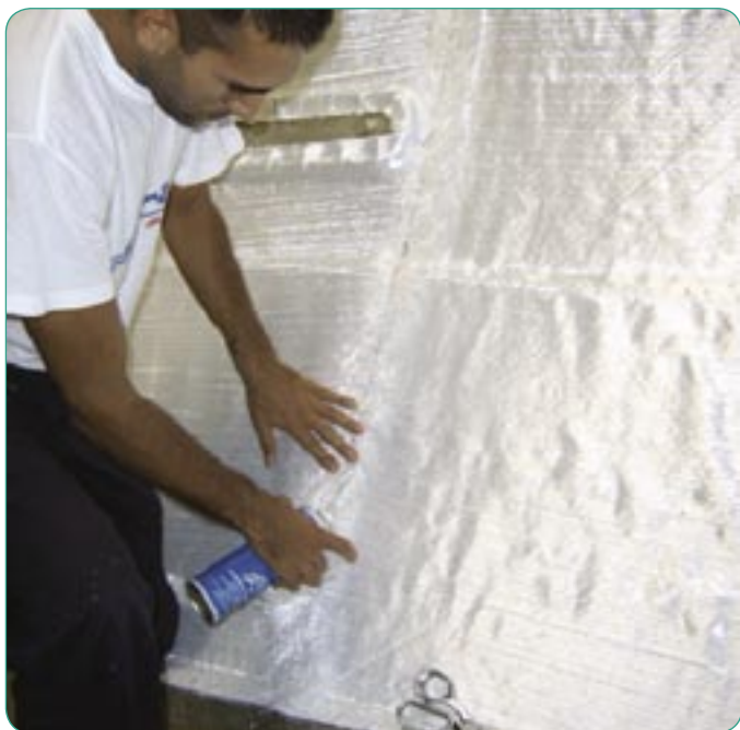
Fig. 7 – Laying up of the dry fibers.
